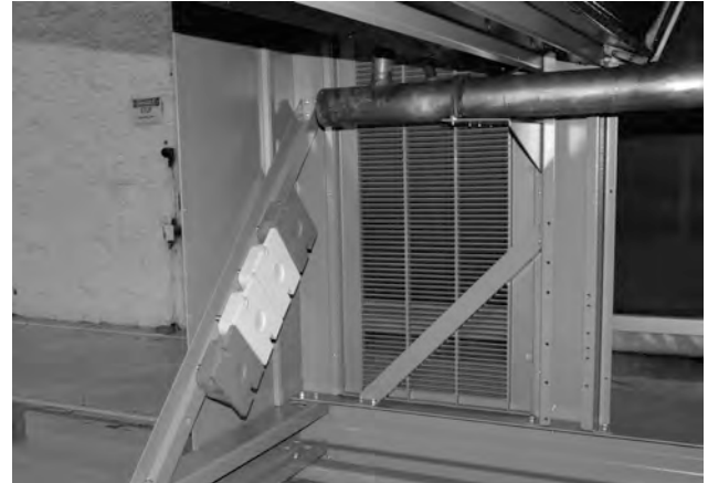
Figure 2. Elastomeric isolators attached for shipping
