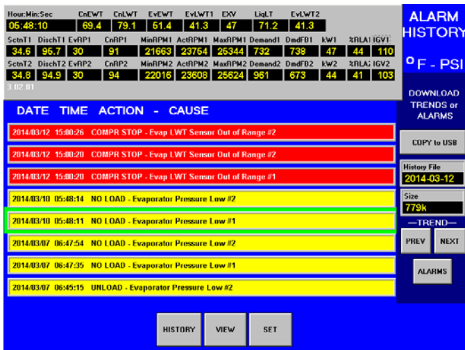
Figure 51: Alarm History Screen with Alarm Detail
